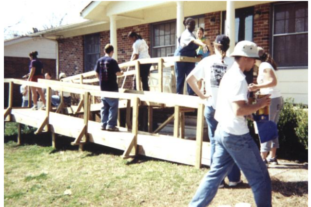
CASA volunteers painting a new ramp
